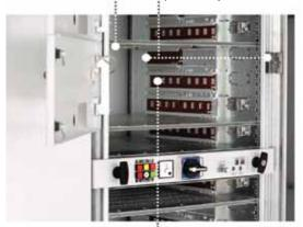
Conductors of the field distribution bus bar
